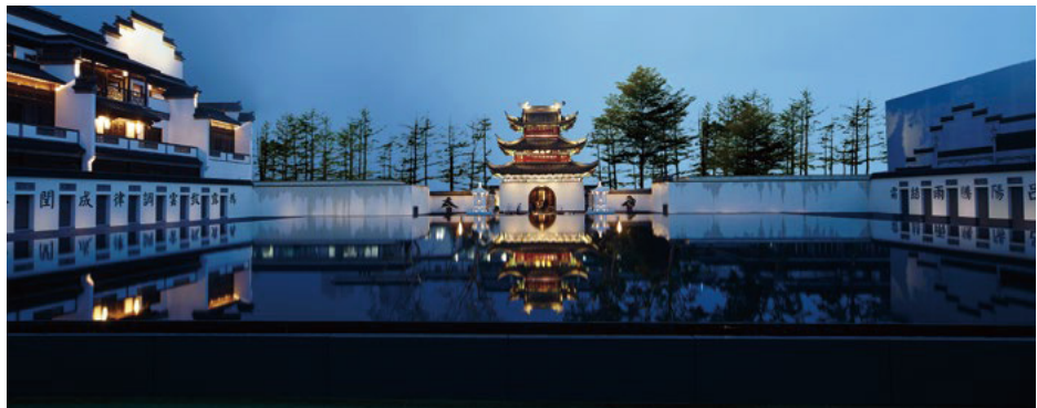
Facade & Landscape Lighting
